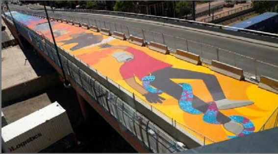
El Paso Chihuahuas - Pedestrian Bridge coating
