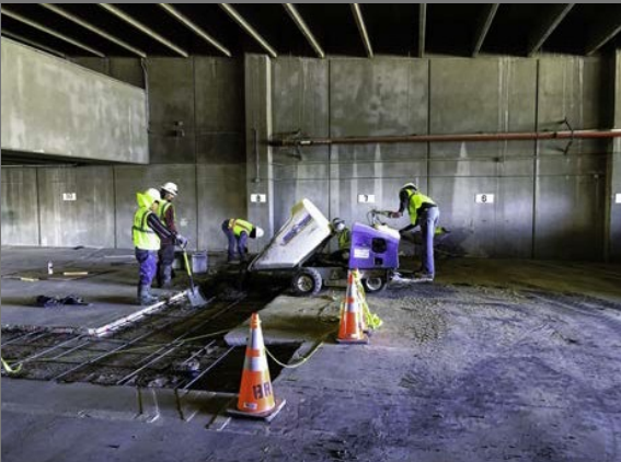
GSA - Replacement of Domestic Water & Sanitary Waste Lines at RC White Building - El Paso, TX
