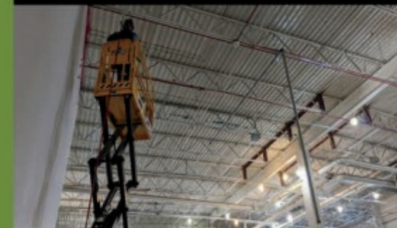
USACE - DESIGN - BID - BUILD B1717 FREEZER CONSTRUCTION AT FORT BLISS
